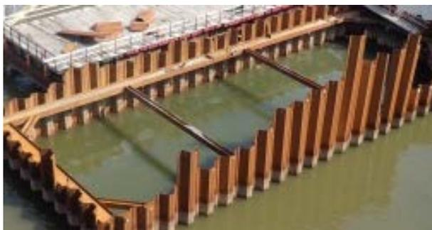
**Typical Arrangement of Cofferdam with Sheetpiles and Struts**
