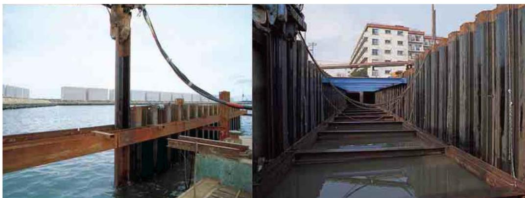
**Installation/Extraction of Sheetpile by Vibratory Method**
